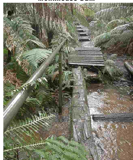
Clark Creek Bridge
